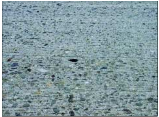
Figure 2. Route 101 surface after diamond grinding.
