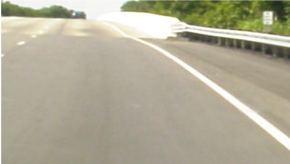
Figure 1. Approaching bridge northbound right lane.
