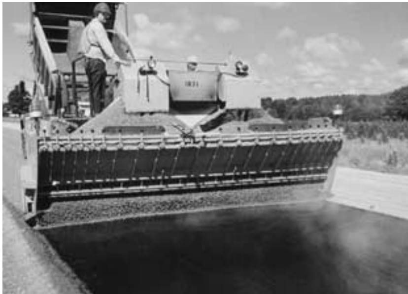
Chip seal operation addresses pavement surface defects on flexible pavement.
