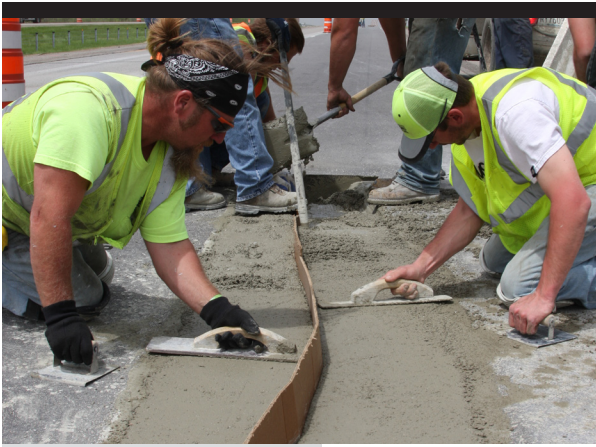
PDR concrete placement operation
