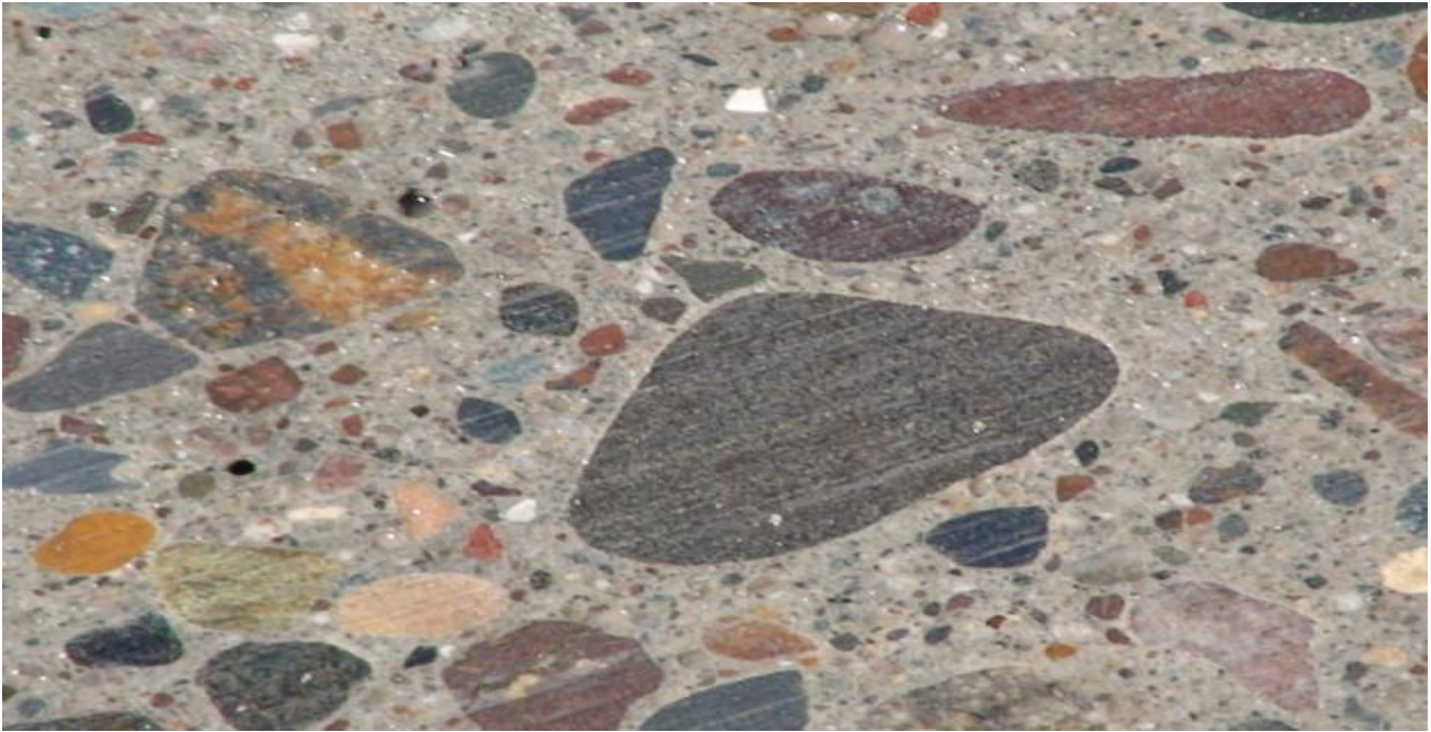
Figure 3: Photo of Flush Grind Immediately After First Pass of Two Pass NGCS Operation
