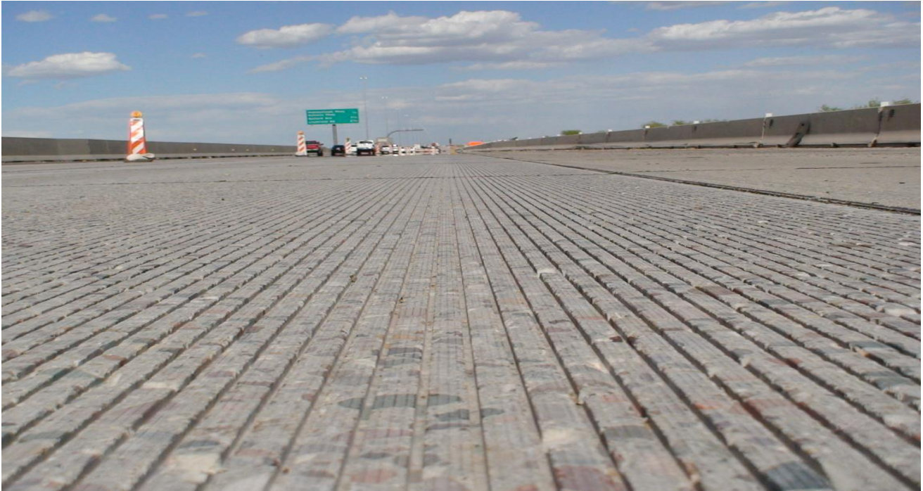
Figure 1: Overall View of NGCS Texture
