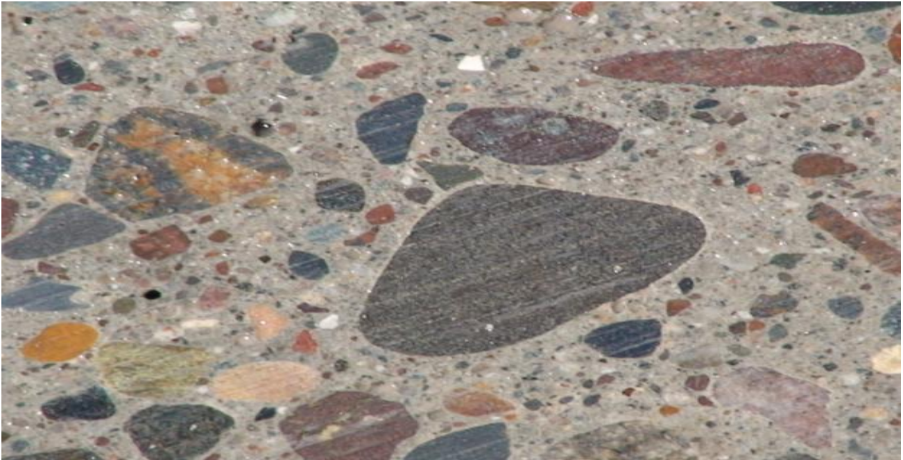
Figure 3: Photo of Flush Grind Immediately After First Pass of Two Pass NGCS Operation
