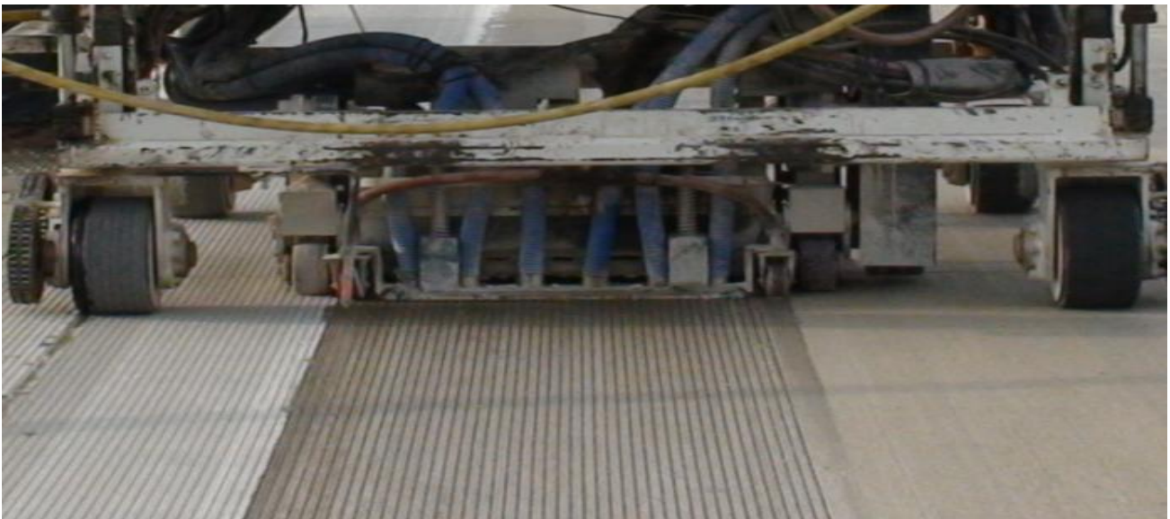
Figure 4: Photo of Grooving Operation of a Two Pass NGCS Operation
