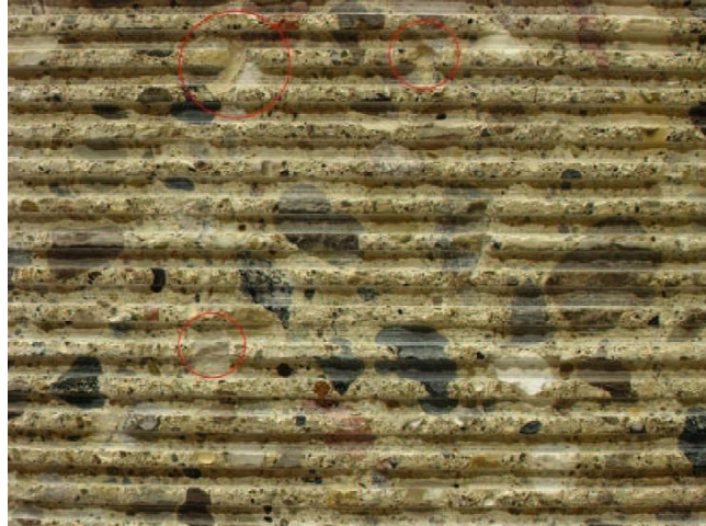
Figure 8 Photo of Breakouts in Fins/Lands During Purdue Testing
