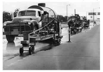
device similar to a grooving machine that could be used to plane and texture hardened pavement surfaces. These devices were used on a number of different concrete applications beginning in the late 1950s, including runways, roadways and dam spillways. In 1962, the first dam spillway was ground at the Indian Valley dam north of Sacramento, CA.
