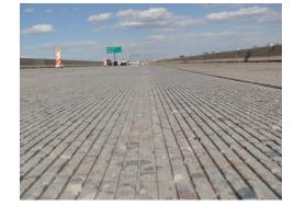
Keeping the environment in mind, a new process called "Buried Treasure" was been developed, where an aging asphalt overlay is removed from an otherwise structurally sound concrete pavement. The reclaimed asphalt is sold or stockpiled for future use with its value used to offset the price of repairs and the diamond grinding of the underlying pavement as a final surface. A truly sustainable process when viewed from an environmental perspective.
