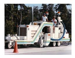
The 1980s was a time that saw technical advancements in both blade and machine development. The Target Company had developed their second generation of grinders and 1983 was the year that Cushion Cut, Inc. unveiled their new PC 5000 production grinding machine. By this time, approximately 5,000,000 sq. yds. of pavement had been diamond ground in the US.
