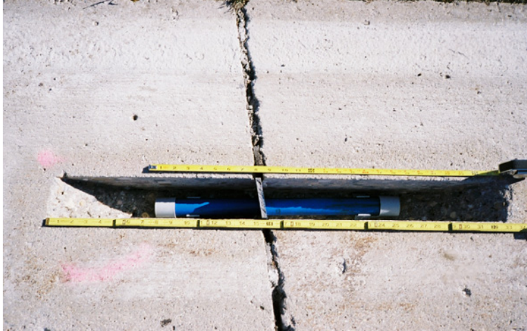
Figure A.4. Proper slot length
