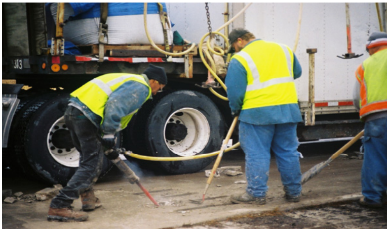
Figure A.3. Slot material removal
