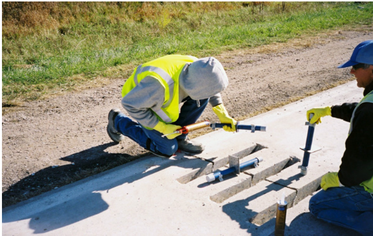
Figure A.5. Dowel chair anchoring
