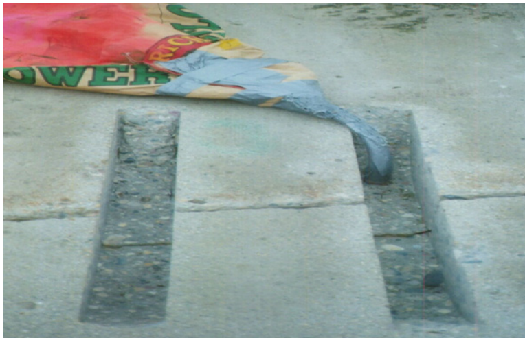
Figure A.6. Plaster crack sealing
