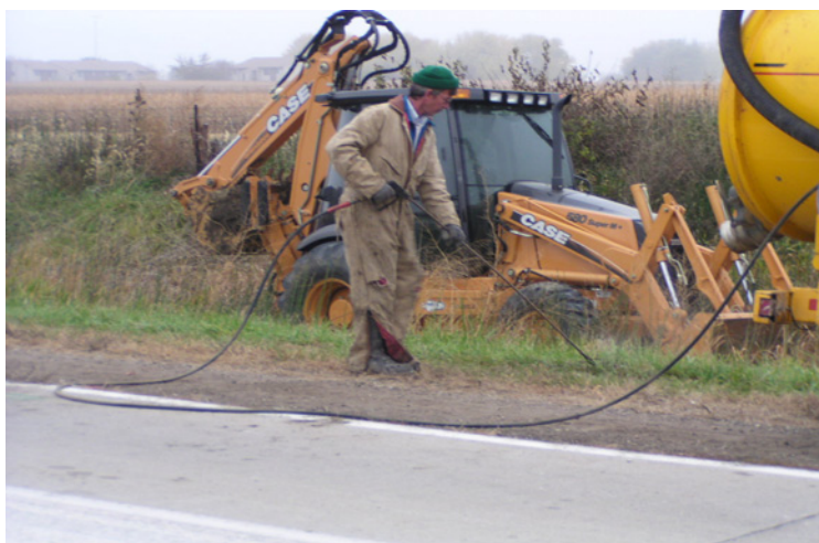
Figure A.9. Instrumentation trench jetting
