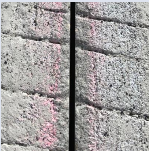
Figure 4 Photo of Media Blasted Joint
