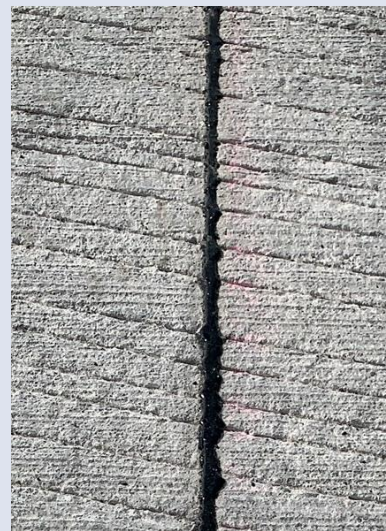
Figure 5 Properly Filled Narrow Joint
