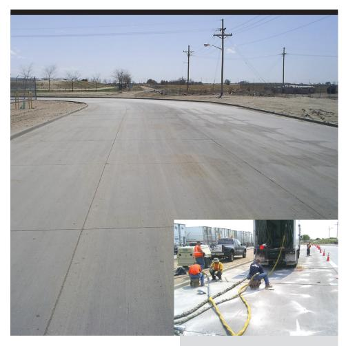
Deep sub-surface voids under pavement corners and joints in areas of utility cuts required deep stabilization, which posed a challenge on this project. These weak sub-grade areas were treated and stabilized without removal of any pavement, using the Uretek USA technology. In addition, seasonal temperatures delayed some of the joint sealing and tighter joints were difficult to lift and align.
