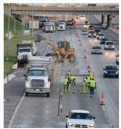
Due to the high level of traffic and poor road conditions, a fast yet long-term solution was needed. DBR, diamond grinding, joint sealing, selective panel replacement and base repair were used on the project for all lanes in both directions.
