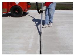
7 Seal cracks and reseal transverse joints.
