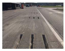
1 Cut slots. (Typically, two to four slots are cut across a joint or crack, parallel to the centerline in the primary wheel paths.)
