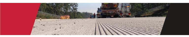
NASA did extensive research in the 1960s and 70s on aircraft hydroplaning and concluded that transverse grooving was superior to longitudinal grooving on runways for water removal and hence hydroplaning prevention. Simply put, the transverse direction has a shorter path for the water to travel to get out from beneath the tire contact patch. Full scale testing with actual aircraft was conducted in that effort.
