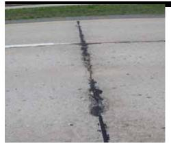
Spalling at transverse joint – location to be repaired with partial depth repair techniques.
