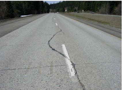
FIGURE 7 Failed longitudinal tape resulting in longitudinal cracking.
