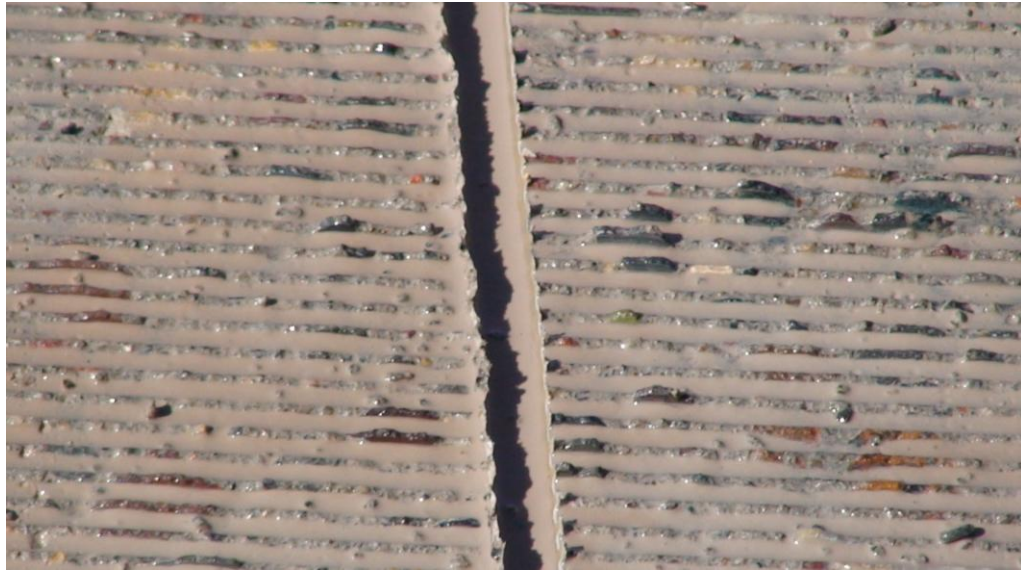
Figure 12 Silicone Sealant Extending Above Surface after Grinding
