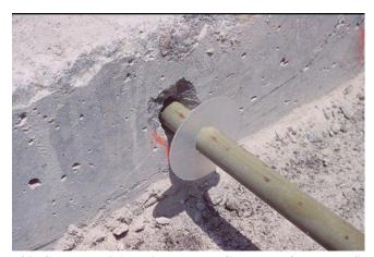
Figure 22. Grout retaining disk. (Photo Courtesy of Mark B. Snyder)
