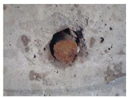
Figure 17. Poor anchoring of dowel into hole that resulted in faulting of the transverse FDR joint. (Photo Courtesy of Mark Snyder)
