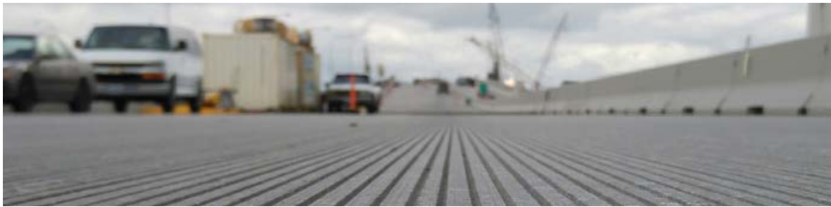
Figure 5: View of longitudinal bridge deck grooving (IGGA, 2020)
