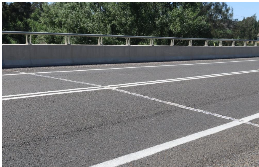
Figure 3: View of concrete deck with sprayed seal surface finish
