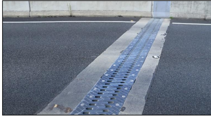
Figure 2: View of the completed waterproofing and asphalt treatment of a bridge deck with the concrete supporting and protecting the expansion joint
