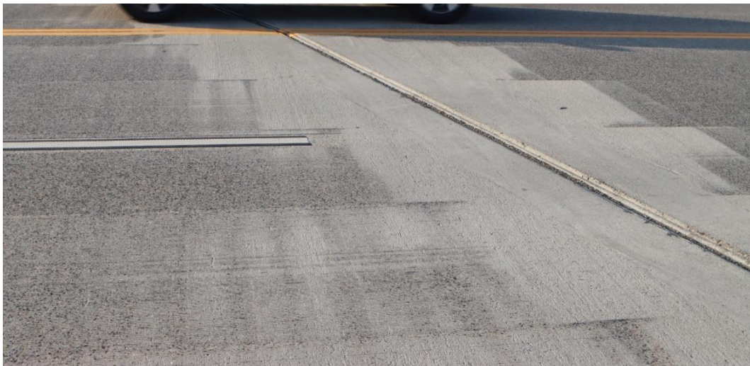
Figure 9: A view of the CDG surface on a new bridge deck in Minneapolis, Minnesota
