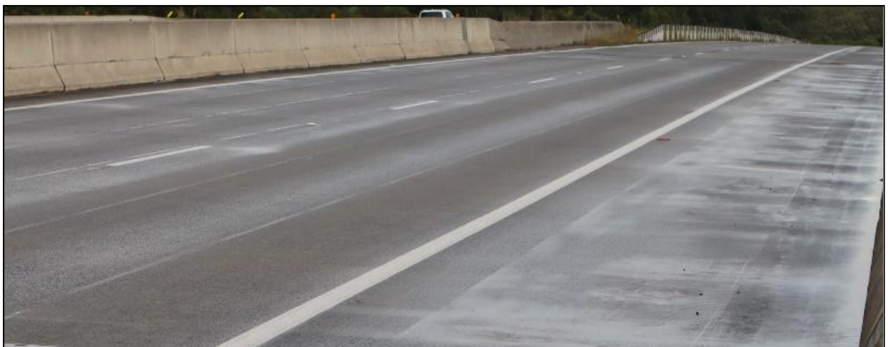
Figure 7: View of narrow overlapping grinding passes and feathering in the kerbside shoulder
