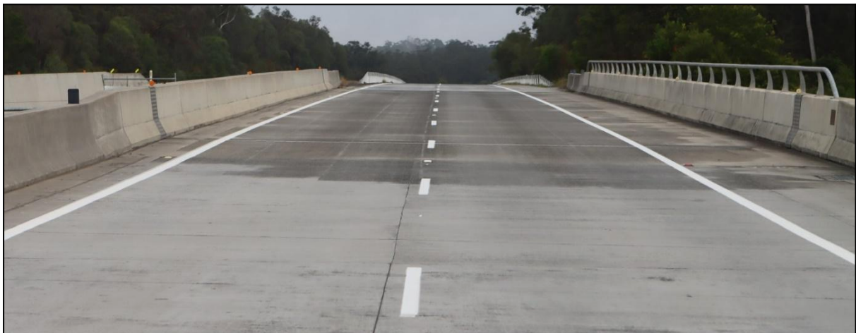
Figure 4: View of CDG on the 4-span bridge to the SB carriageway of the Pacific Highway, NSW
