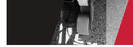
**DOTS ACROSS THE COUNTRY DIAMOND GRIND PAVEMENT** to optimize pavement performance while minimizing their spending, often employing it to smooth out uneven spots in a pavement. They specify bump grinding—that is, grinding restricted to just the uneven areas—in an effort to address only troublesome locations and thereby conserve resources while meeting smoothness requirements. However, when it comes to diamond grinding, this selective approach is not always the most effective one.
