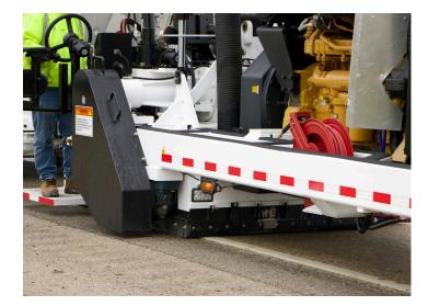
Additionally, when pavement engineers are at the drafting table designing new, heavily phased paving projects, they should anticipate a significant amount of bump grinding and thereby consider incorporating continuous diamond grinding over the entire project to obtain the best value and performance from the grinding product.
