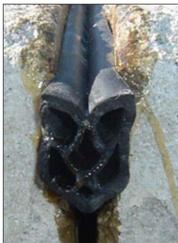
Figure 5 Compression Seal Installed 3
