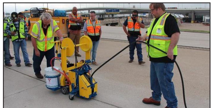
Figure 3 Joint Sealant Installation Equipment
