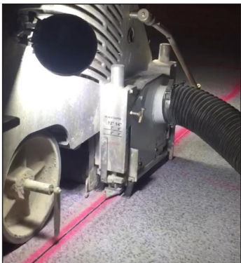
Figure 6 Photo of Early Entry Saw Joint With Vacuum Attachment
