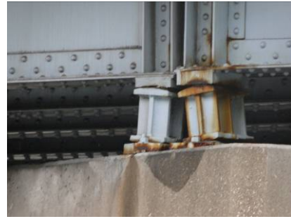
Figures 21 & 22. Tilted rocker bearings during cold weather
