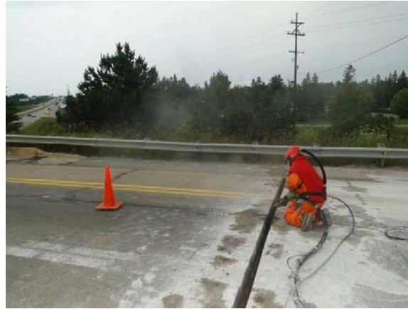
Figure 33. Sandblasting the exposed edges of pavement
