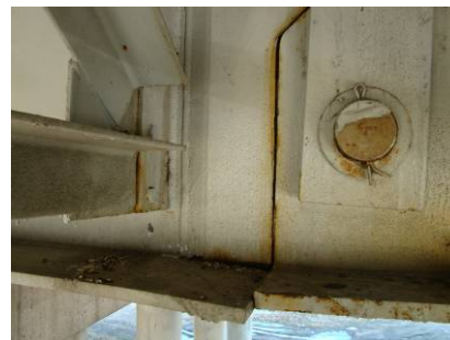
Figures 19 & 20. Pin & Hangers closed during cold weather
