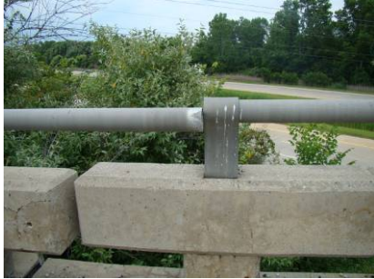
Figures 15 & 16. Aluminum tube rail separation
