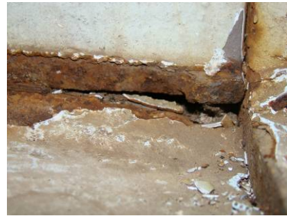
Figures 23 & 24. Examples of damage from beam end contact
