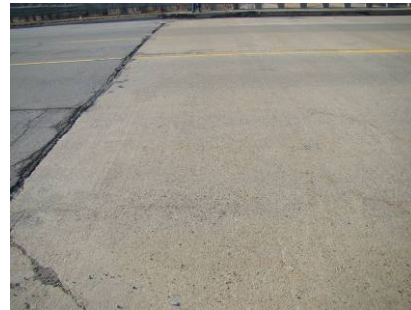
Figures 17 & 18. Diagonal deck cracks in tailspans
