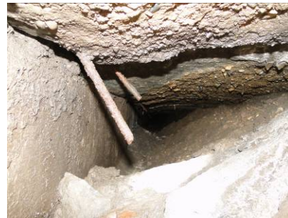
Figures 29 & 30. Approach settlement and void behind backwall
