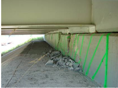
Figures 27 & 28. Dependent backwall delamination and spalling
