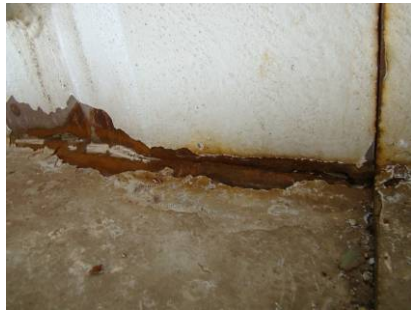
Figures 23 & 24. Examples of damage from beam end contact
