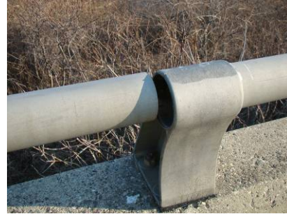
Figures 15 & 16. Aluminum tube rail separation
