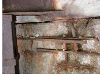
Figures 27 & 28. Dependent backwall delamination and spalling
