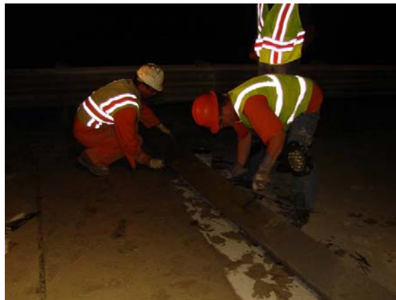
Figure 34. Applying lubricant adhesive to both contacting edges
