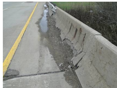
Figures 13 & 14. Crushed concrete railings
