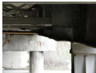
Figure 31. Buckling tailspan beam
