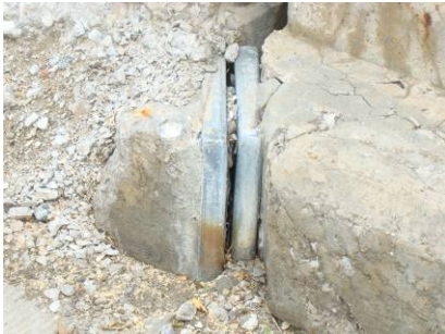
Figures 11 & 12. Expansion joints permanently closed
