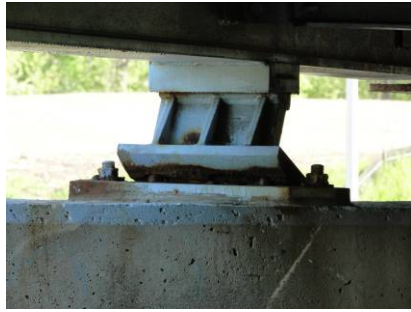
Figures 21 & 22. Tilted rocker bearings during cold weather
