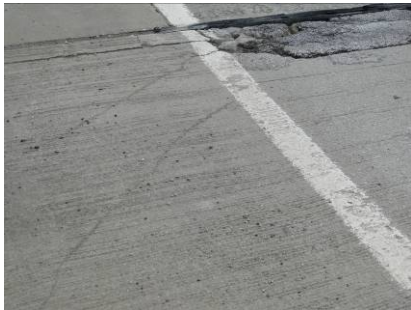
Figures 17 & 18. Diagonal deck cracks in tailspans
