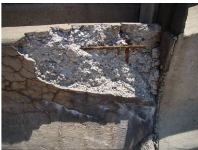
Figures 13 & 14. Crushed concrete railings
