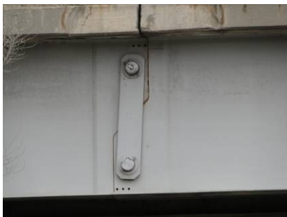
Figures 19 & 20. Pin & Hangers closed during cold weather
