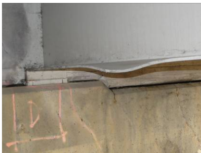
Figure 31. Buckling tailspan beam
