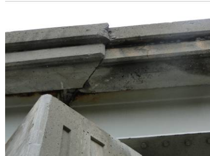
Figures 11 & 12. Expansion joints permanently closed
