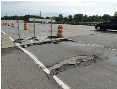
Figures 29 & 30. Approach settlement and void behind backwall
