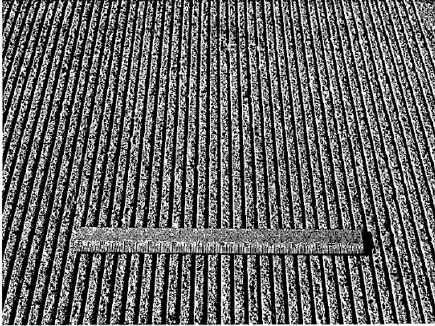
**Figure 7 RWP 1/8" X 1/8" at 1/2" Centers Grooving Pattern<sup>1</sup>**
